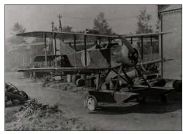
First flight: Autumn 1917 Span: 9.54m/31ft 4ins Length: 7.76m/25ft 5ins Max weight: 897kg/1,978lb Max level speed: 94knots/174kph Power plant: One 150shp/112kW Bentley BR 1 rotary
